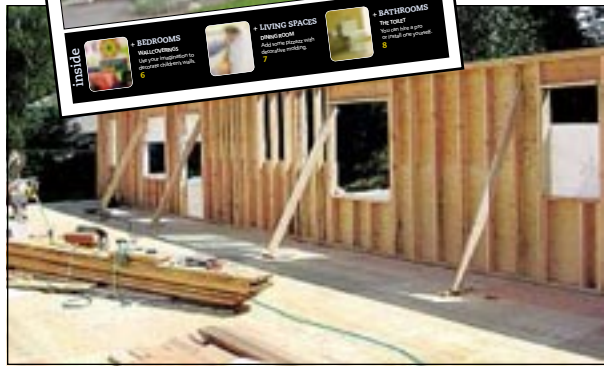
On the Spot begins work on an add-a-level in North Haledon.
