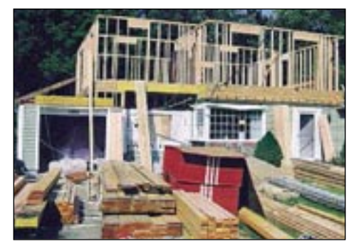
The GTFM crew frames out a 1,200-square-foot second level.
