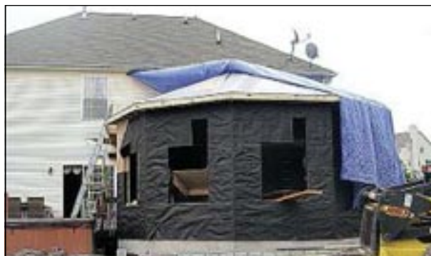
An add-on in Lafayette by On the Spot, in progress.
