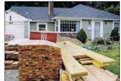
A ranch house in Wyckoff awaits a new level by GTFM.
