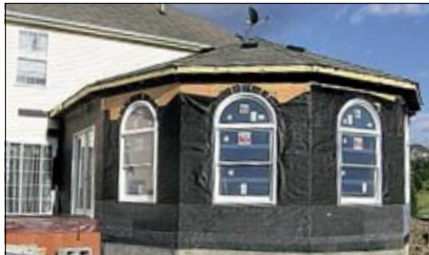
New roofing and windows completed.
